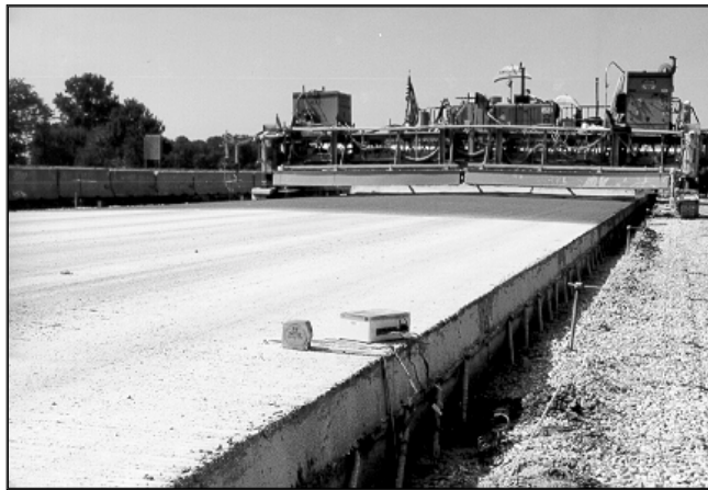
Figure 2. Typical application of maturity method in the field. Note maturity meter in the foreground with three thermocouple wires inserted into the pavement at different depths.
