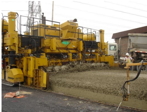
Figure 2: Typical casting of concrete for CRCP
