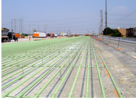
Figure 1: Typical reinforcing layout for CRCP
