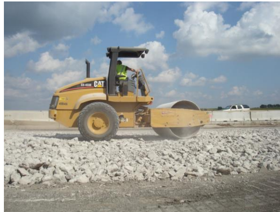
Figure 7: Compaction of sub-base using roller
