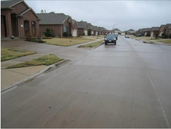
a) ICC slabs in residential area
