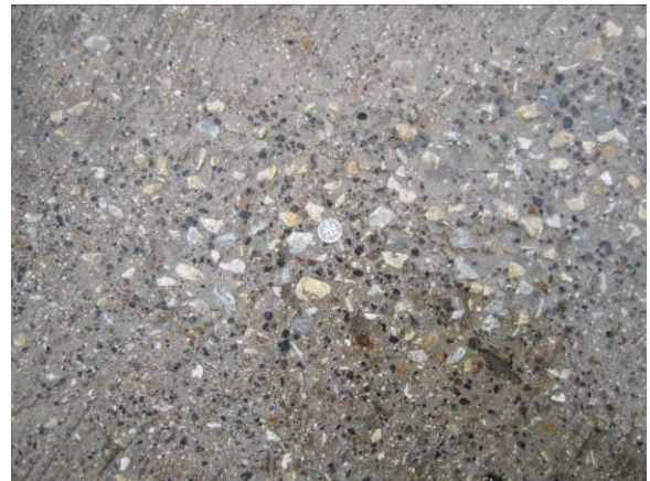
d) ICC pavement surface
