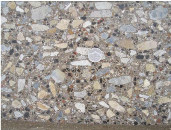
c) Sawed surface of ICC along curbs
