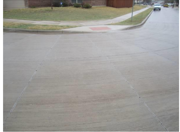
b) ICC slabs along horizontal curve
