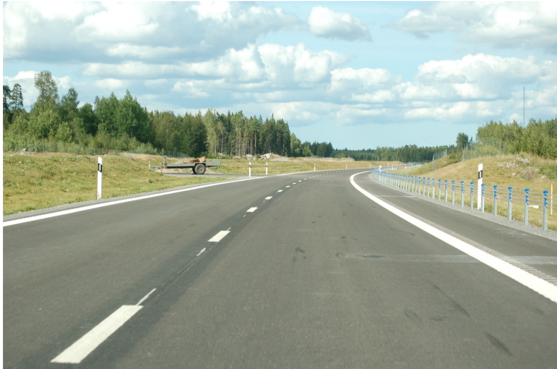
Figure 3. The AC test site on highway E4.
