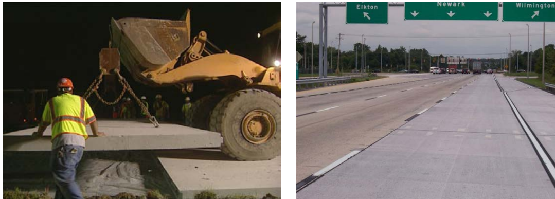
Figure 3. Installation of a precast panel for the DelDOT project (left) and completed project (right). (Photos courtesy of Delaware DOT)
