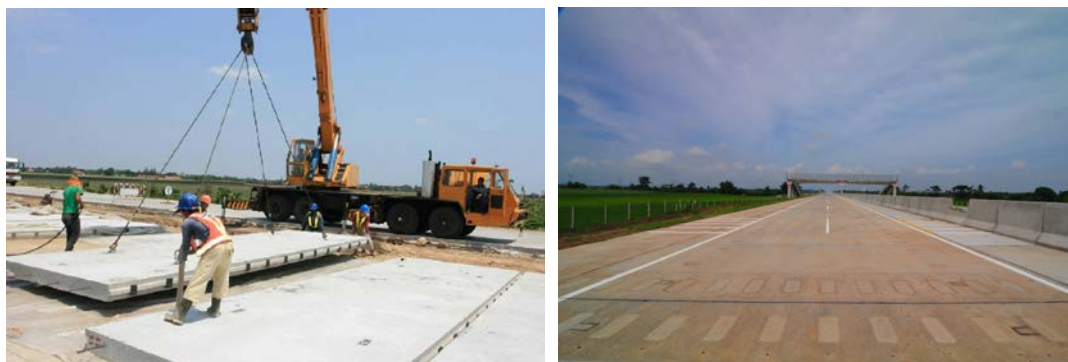
Figure 4. Installation of PPCP panels and a section of finished pavement in Indonesia (photos courtesy of Tommy Nantung)
