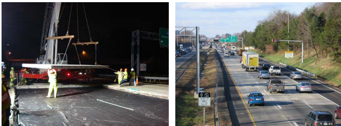
Figure 5. Installation of a precast panel for the Virginia project (left) and the completed pavement after opening to traffic (right).
