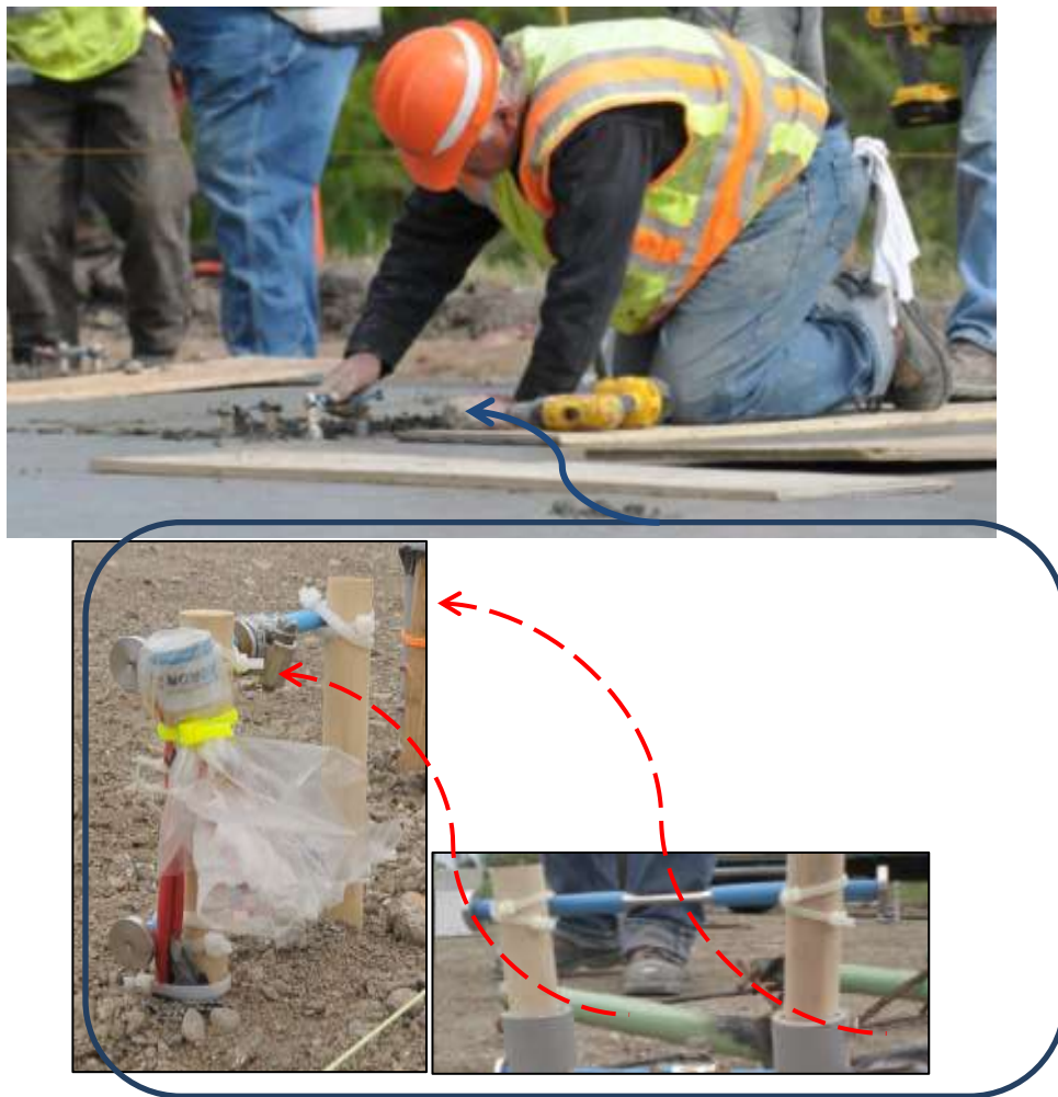
Figure 7. Technique for installing the static strain gage in the upper concrete layer for Cells 71 and 72.
