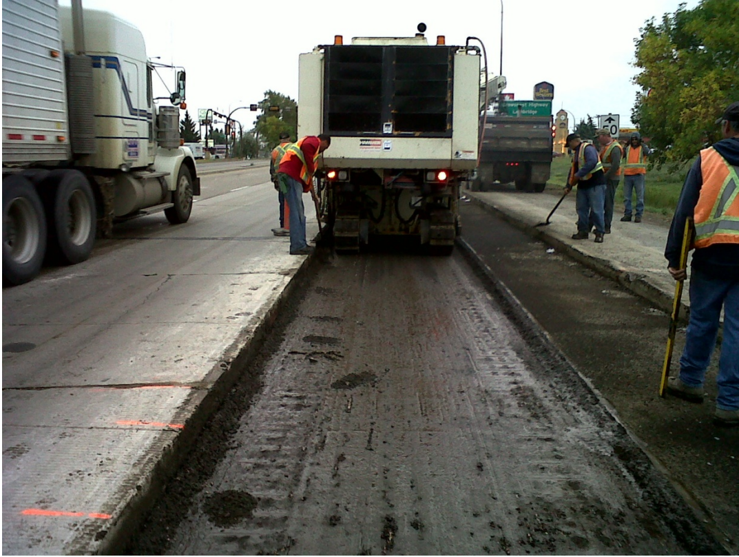
Figure 4. Milling of asphalt beneath concrete pavement
