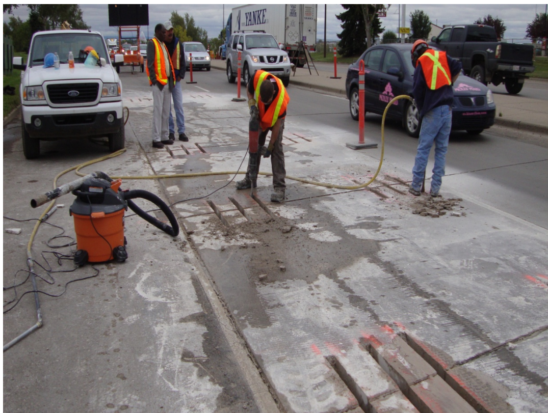
Figure 6. Saw cuts and jack hammering for the dowel bar retrofit
