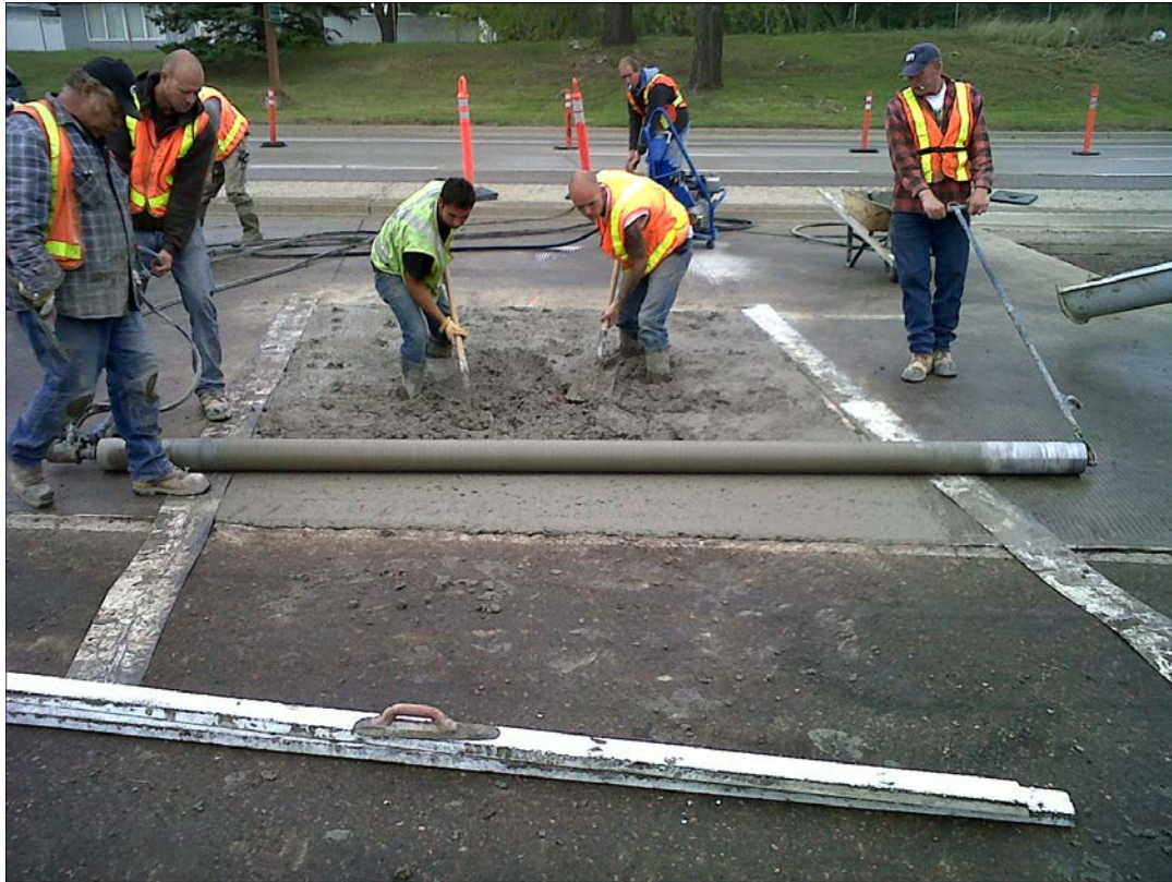
Figure 5. Power roller screed for concrete finishing
