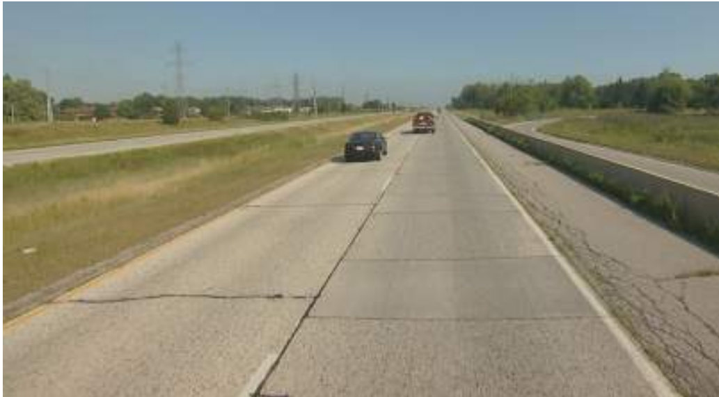
Photo 1. Recent Photo on Northbound Lanes
