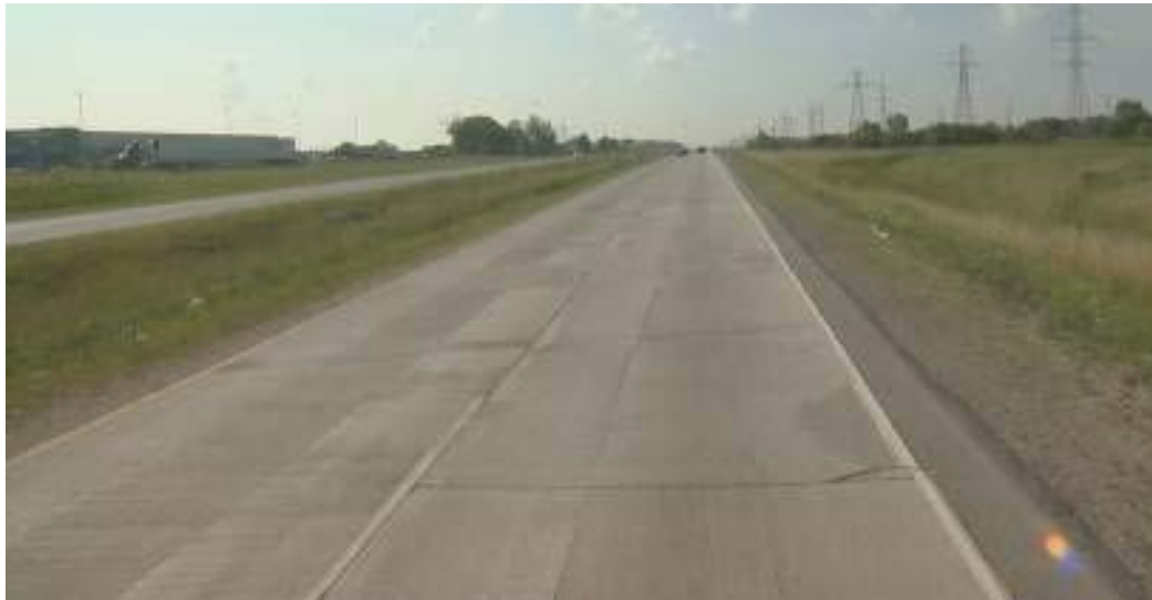
Photo 2. Recent Photo on Southbound Lanes
