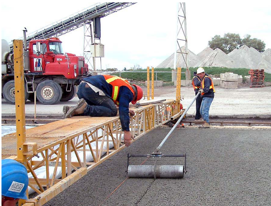
Figure 3. Transverse Joint Rolling (Trial Slab)
