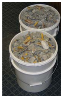
Figure 5. Example of spall fragments collected from new runway and taxiway pavements at Airbase A.
