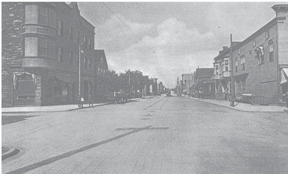
FIGURE 6: Northerly view of 6 th Street, showing newly finished granitoid pavement, reproduced from circa 1910 advertisement brochure (51).
