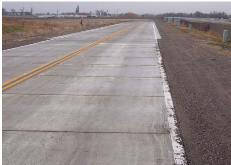
Figure 3. Photograph of Cell 32 (foreground) in 2003, looking southeast (image courtesy of the Concrete Paving Association of Minnesota).
