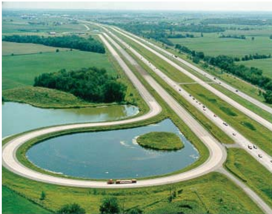
Figure 1. Aerial photo of MnROAD (image courtesy of Minnesota Department of Transportation).
