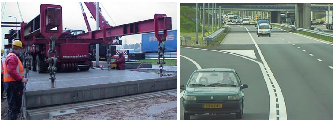
Figure 5. The ModieSlab technology in tests section along A50 and A12 in Netherlands.
