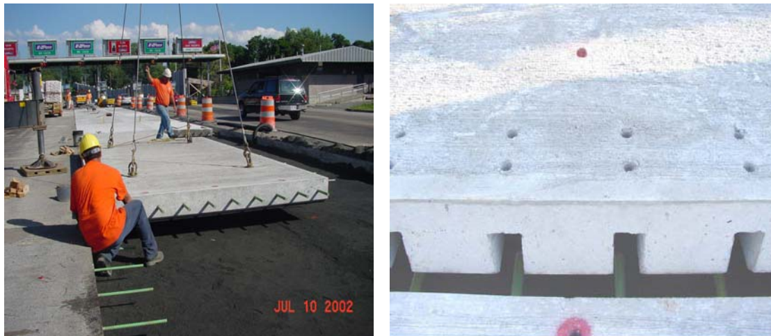
Figure 2. The Super Slab System
