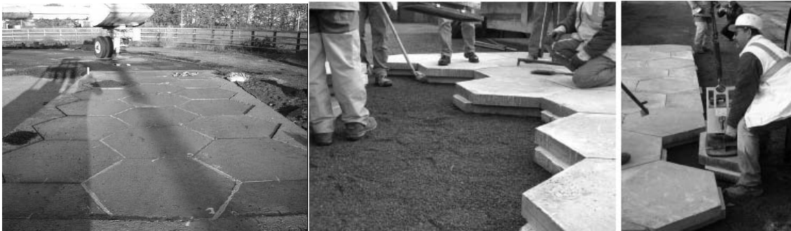
Figure 8. Installation of keyed hexagonal slabs in France
