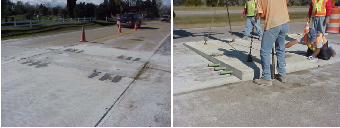
Figure 7. The full depth precast repair system (M-25, MI)
