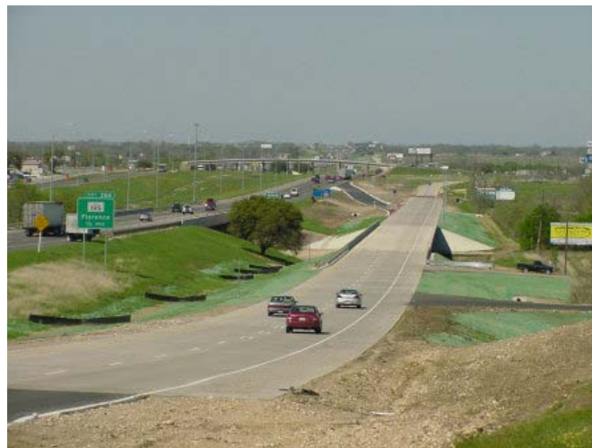
Figure 1(b). Completed project along I-35 in Georgetown, TX
