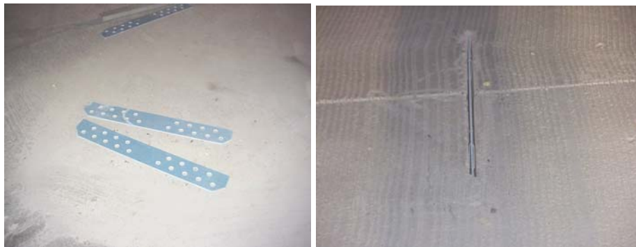
Figure 3 Uretex fiber glass stitches
