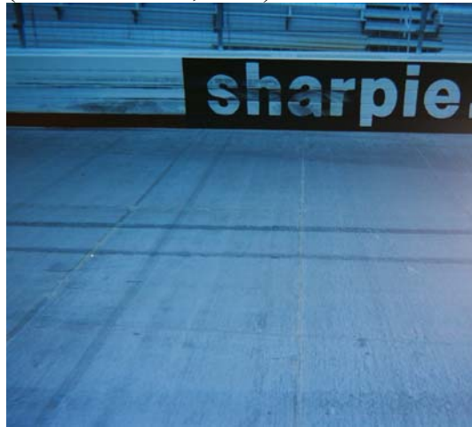
Figure 14b 5 Foot Sawcuts.
