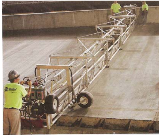
Figure 14a Sawing in the Banked Sections (Gomaco World, 2008)
