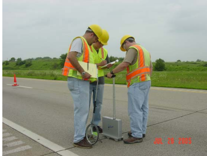
Figure 13- Field trials equipment and set up
