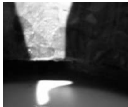
a) Void and Erosion Under the Concrete Slab of Poor Condition Section
