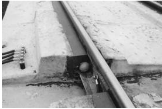
Fig. 14: Embedded rail main line test-section in Waghäusel opened 2001
