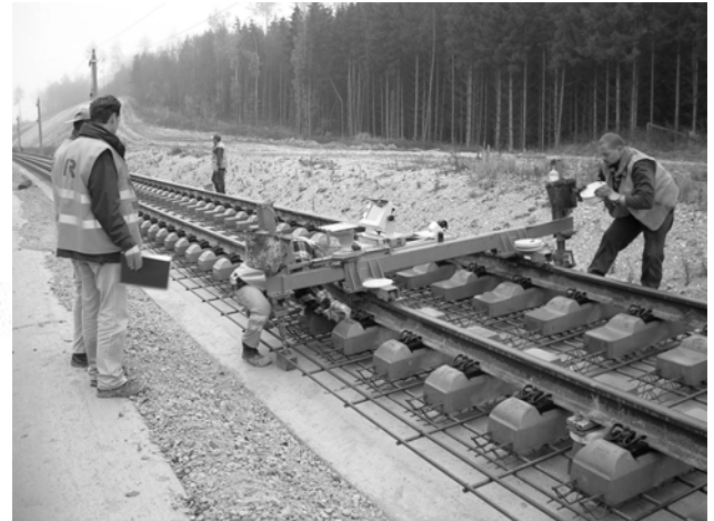
Fig. 8: Final adjustment of the sleeper panel before concreting the CRCP-layer (Highspeed line Nuremberg – Ingolstadt)
