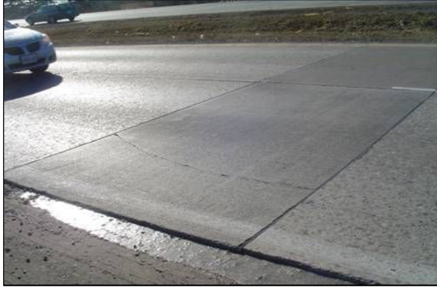
Photo 1. Northbound Lane Full Depth Repair Section
