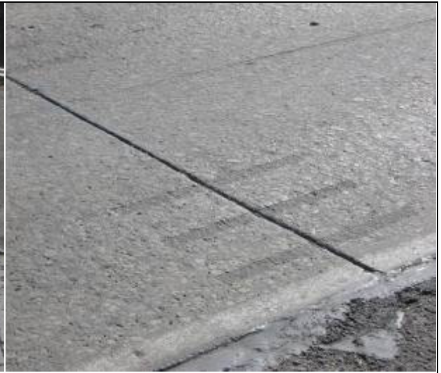
(b) Typical condition of backfill
