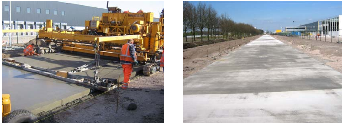
Figure 2 The Tilburg pavement during (left) and after construction (right).
