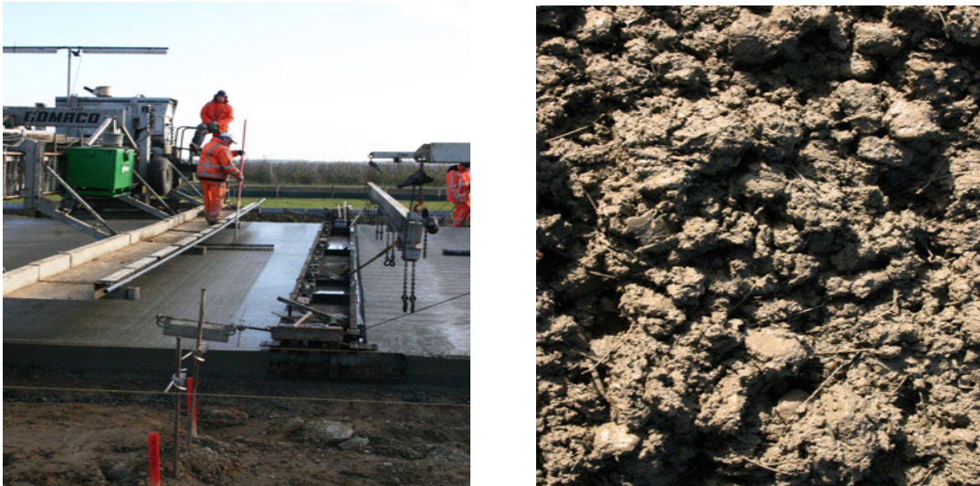
Figure 4 The Roermond pavement during construction and the mix in detail.
