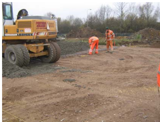
Figure 5 Placing the dowels at the predefined location of a transverse shrinkage joint.
