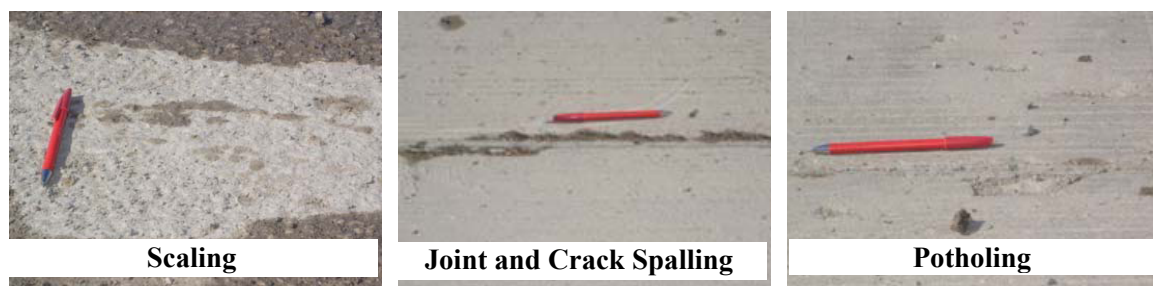
Figure 7. Test Section PCI Photos – Apr. 2, 2008
