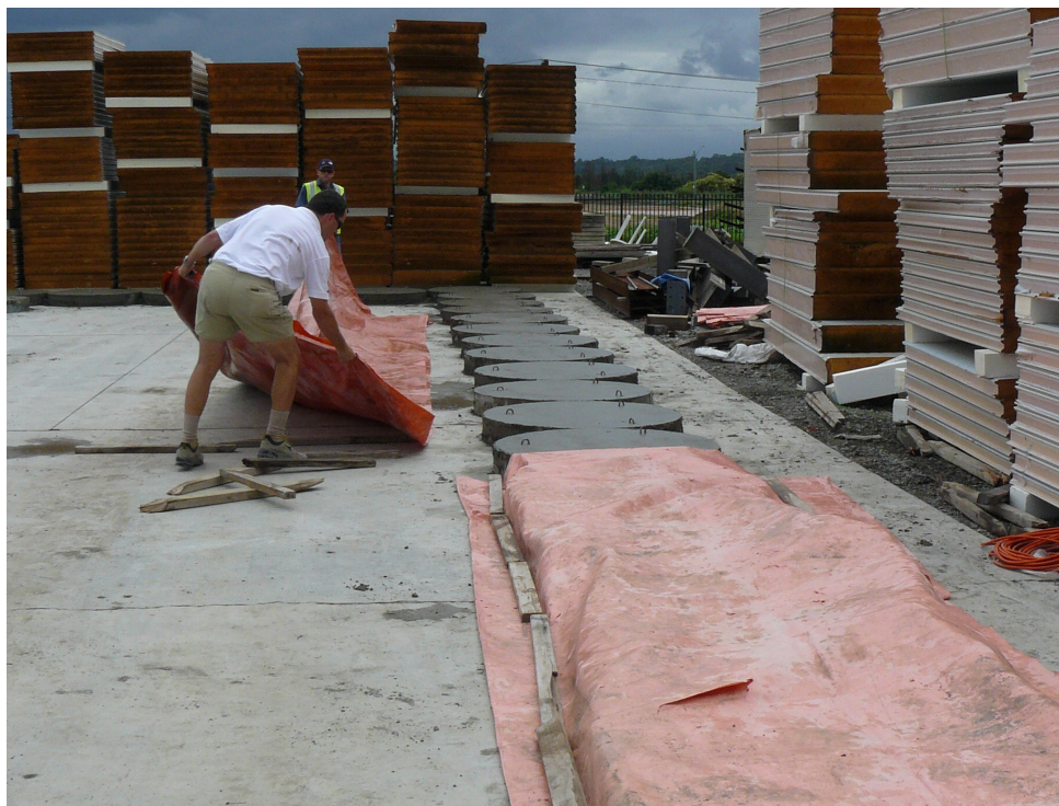
Figure 16 – Curing Preparation (Typical)
