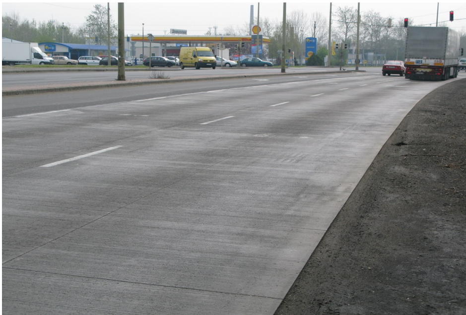
Photo 2 Whitetopping surface with joints (April 2008)
