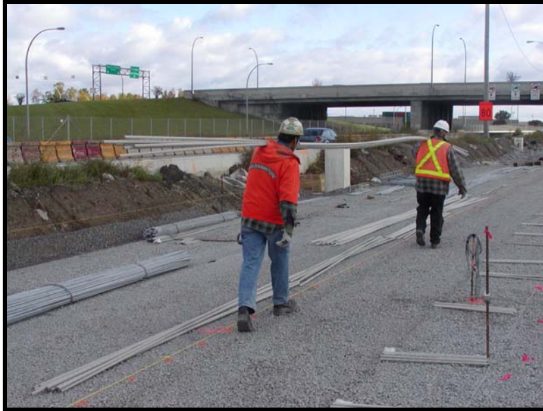
Figure 2 – Handling of GFRP reinforcement bars
