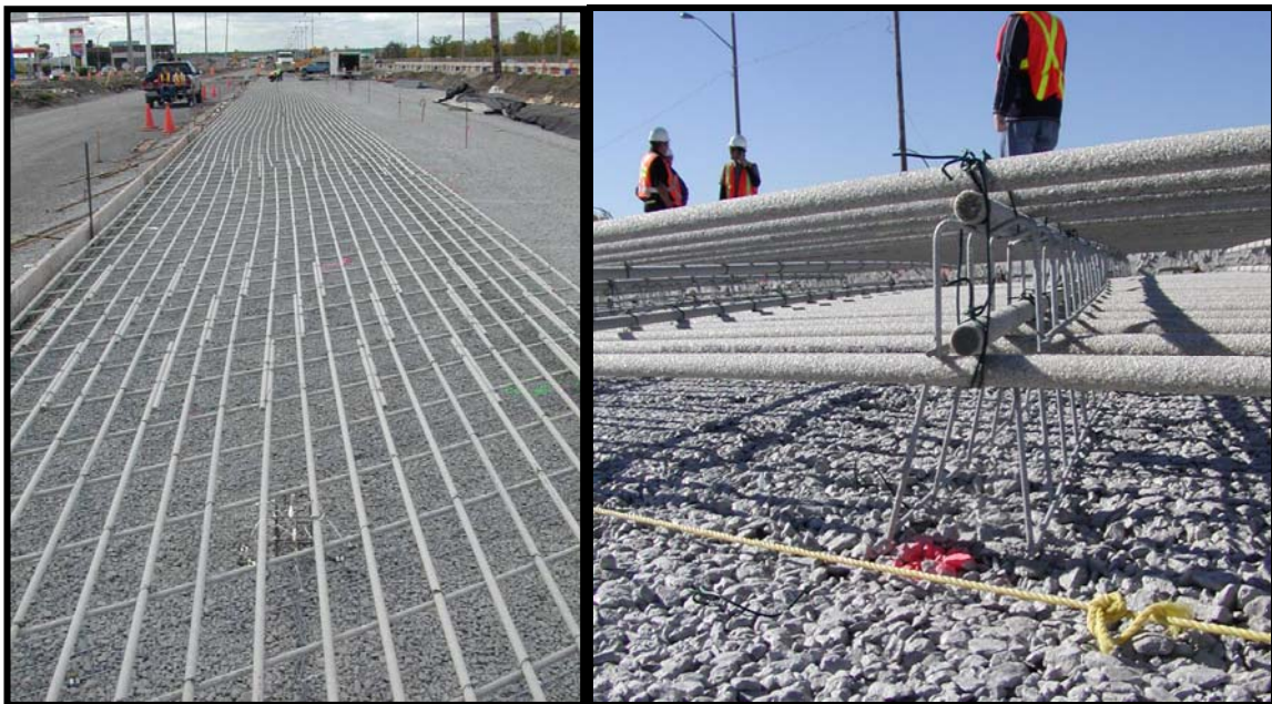
Figure 3 – GFRP reinforcement bars in one layer and 2 layers
