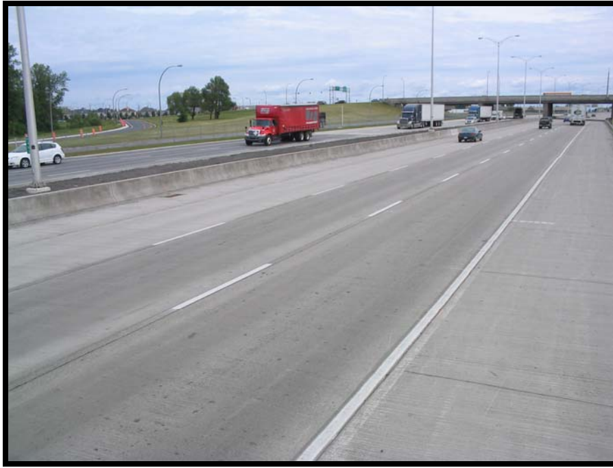
Figure 8 - Overall view for HW-40
