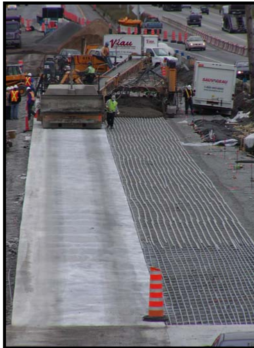
Figure 4 - Casting of the concrete over GFRP bars in left lane
