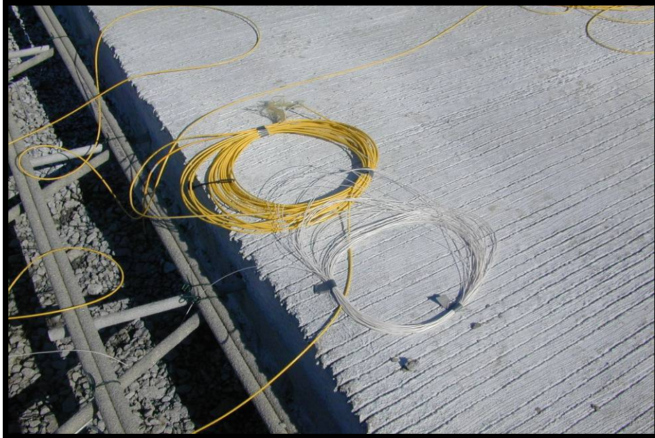
Figure 7 - Fibre Optic Distributed Brillouin Sensors (FODBS)
