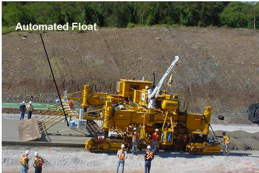
Figure 7. Automated float behind the paver.
