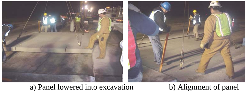
Figure 5. Panel placement process.
