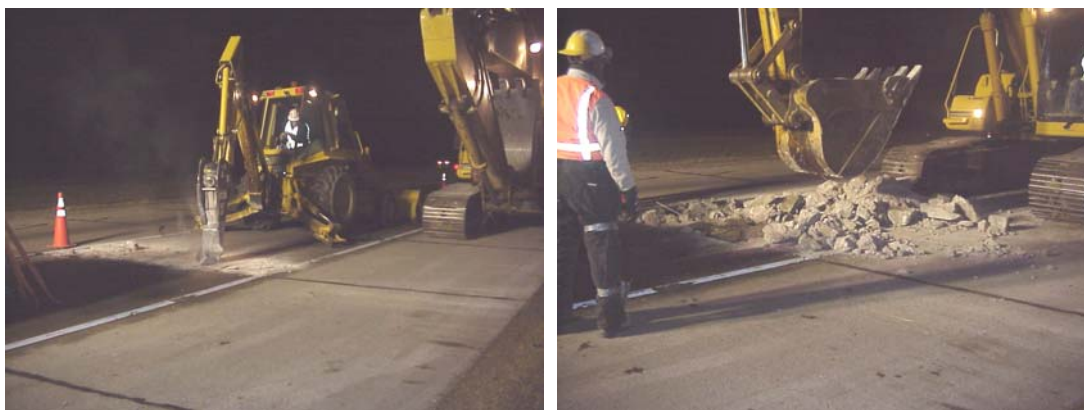
a) Slab demolition
