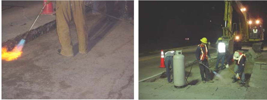
Figure 4. Base preparation activities.
