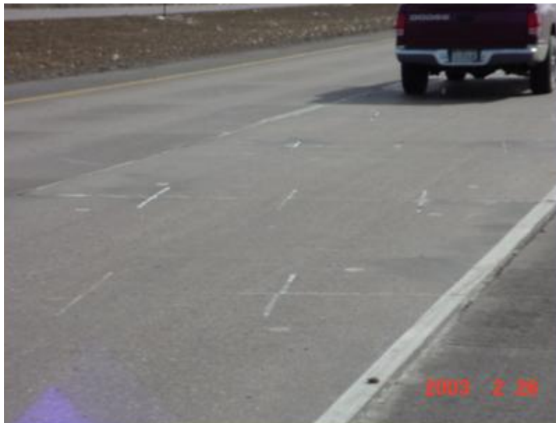
Figure 7. Completed cluster of precast panels.
