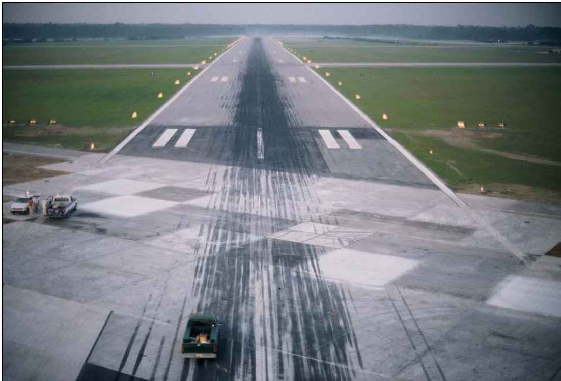
Figure 2. Charleston runway intersection (photo provided by Gary Skoog, HNTB).
