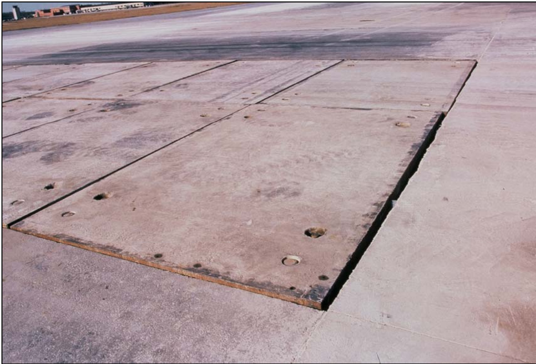
Figure 3. Precast panels in place, Savannah photo provided by Gary Skoog, HNTB).
