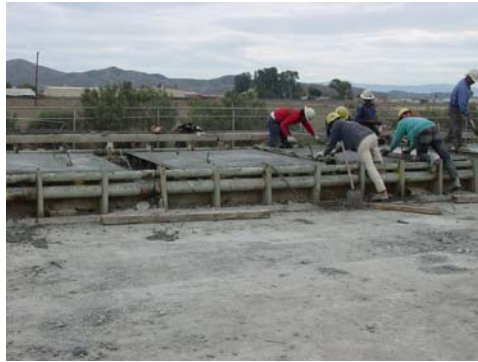
Figure 9. Casting of Two Slabs in Bed
