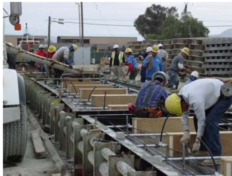
Figure 2. Configuration of Casting Bed
