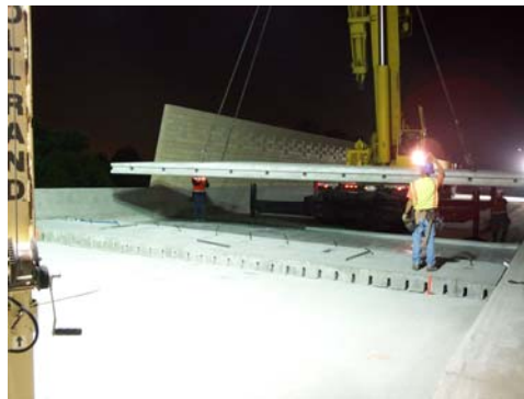
Figure 14. Lean Concrete Base
