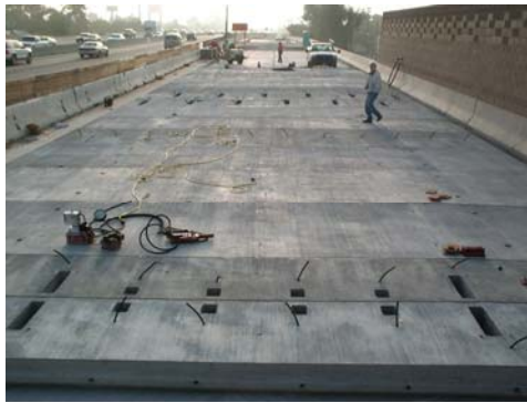
Figure 19. Post Tensioning Operation
