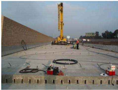
Figure 15. Crane Working Behind Temporary Barrier
