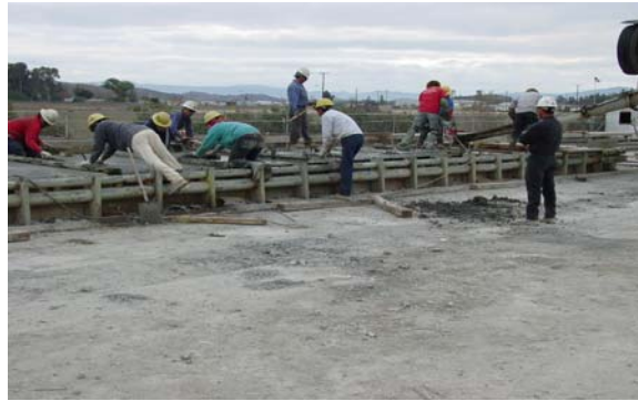
Figure 11. Casting Slabs
