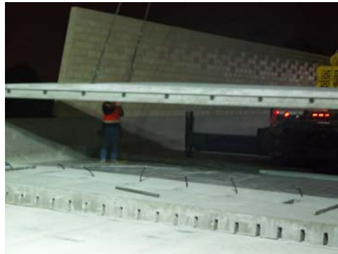
Figure 18. Placement of Slabs
