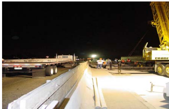
Figure 16. Unloading Slabs From Truck
