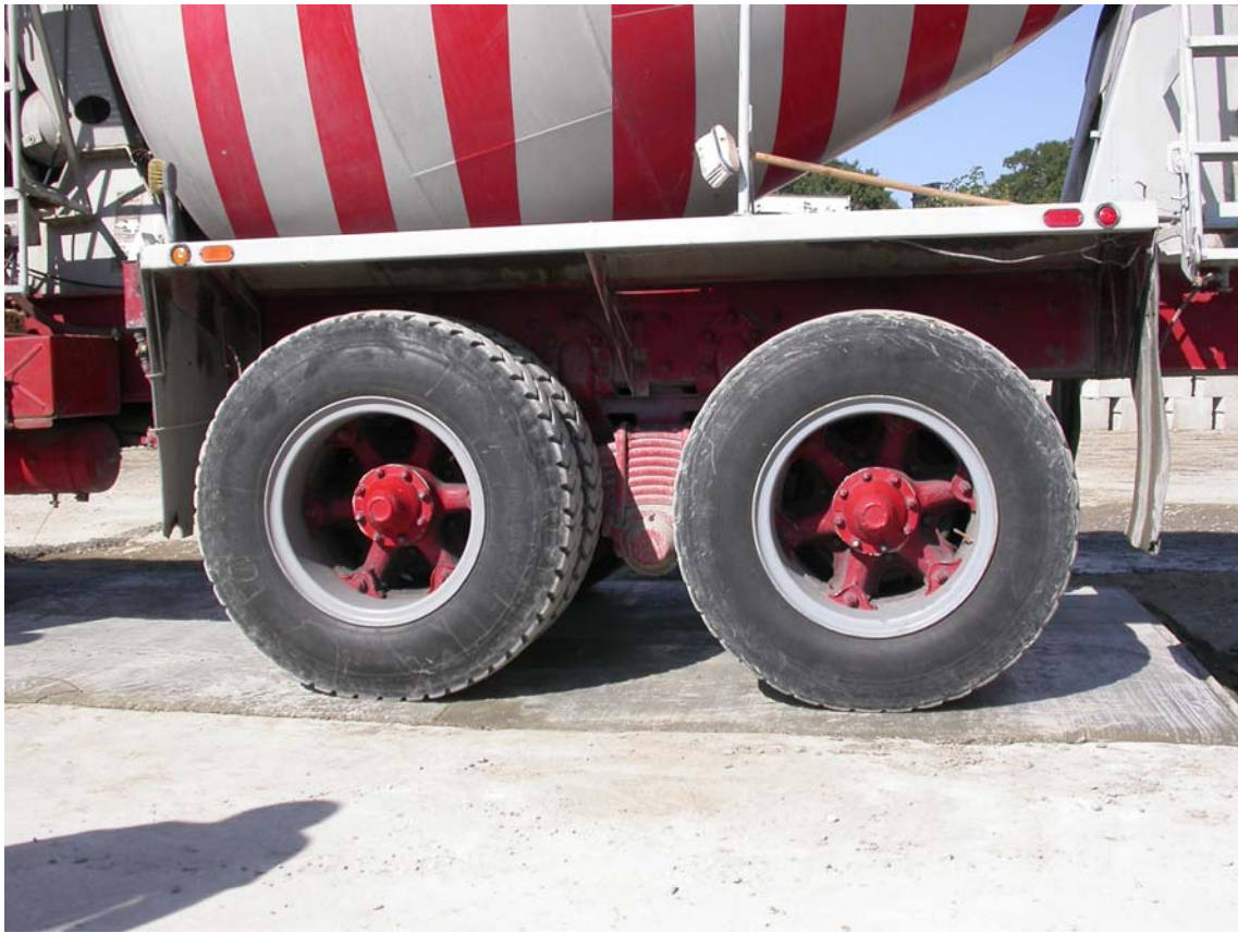
Figure 7: NHESC supports a ready mix truck in only 4 hours after placement
