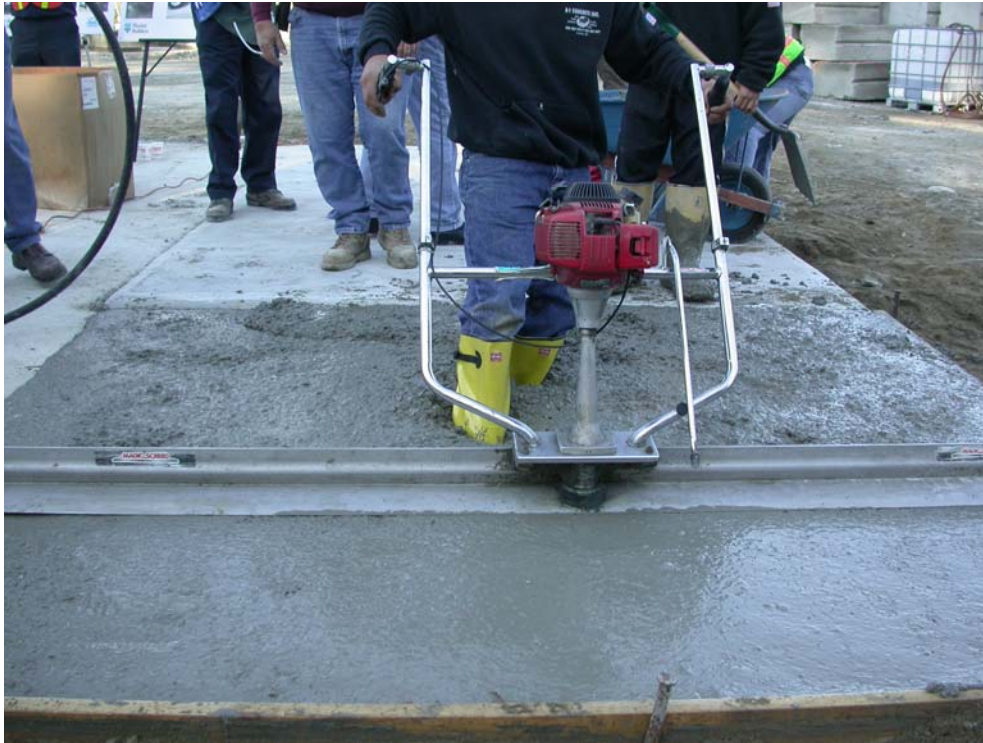
Figure 3: NHESC is leveled using a vibratory screed
