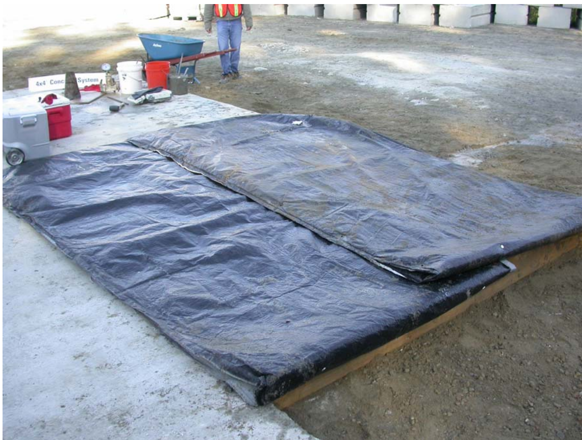
Figure 4: Curing the NHESC using an insulating blanket.
