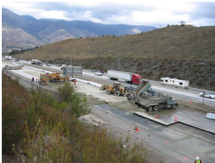
Figure 4. Paving operation on construction roadbed and counter-flow traffic with QMB on traffic roadbed
