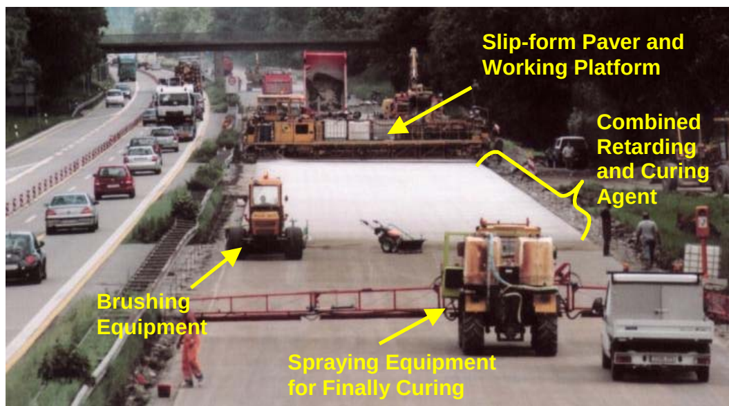
Figure 7. Construction of a concrete road pavement with “Austrian exposed-aggregate concrete surface”: Concrete placement with slip-form paver, spraying with a combined retarding and curing agent from a platform (light shade), brushing off the unhardened surface mortar, and spraying with a customary curing compound from a separate carrier.
