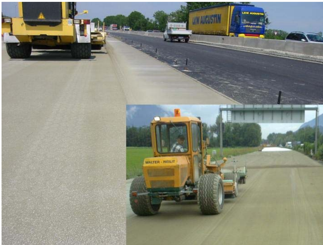
Figure 8. Construction of a concrete road pavement with “Austrian exposed-aggregate concrete surface”: Brushing off the unhardened surface mortar.
