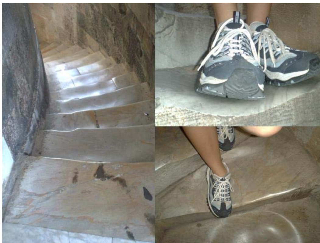
Figure 3. Old stairs of stones with little resistance to polishing, were heavily polished over centuries by pedestrian traffic only, show the importance of a high PSV value of the aggregates for skid resistance of our roads with heavy traffic loads.
