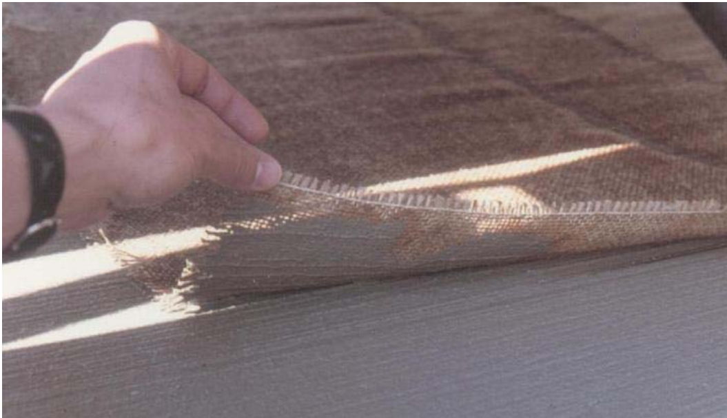
Figure 5. A piece of burlap is dragged along the green concrete from a platform; the longitudinal texture produced by this ensures a high skid resistance and little noise development of the concrete road.
