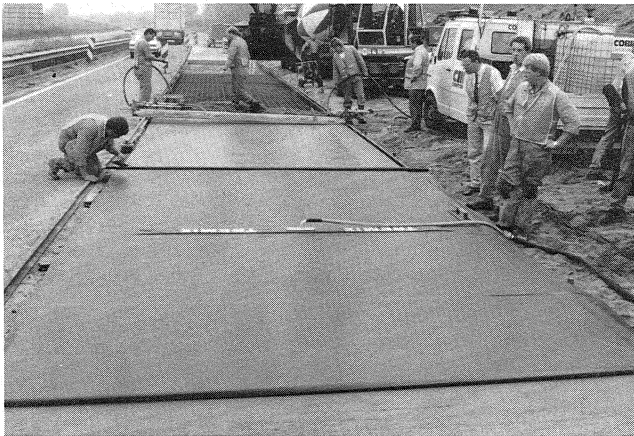
figure 8: Suction mat is placed
