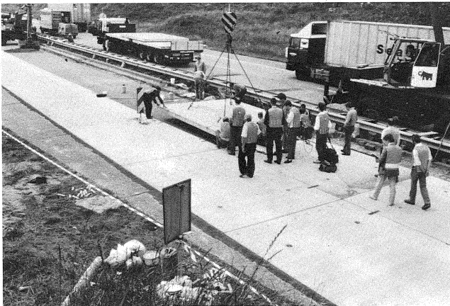
figure 11: A prefabricated slab is placed into position
