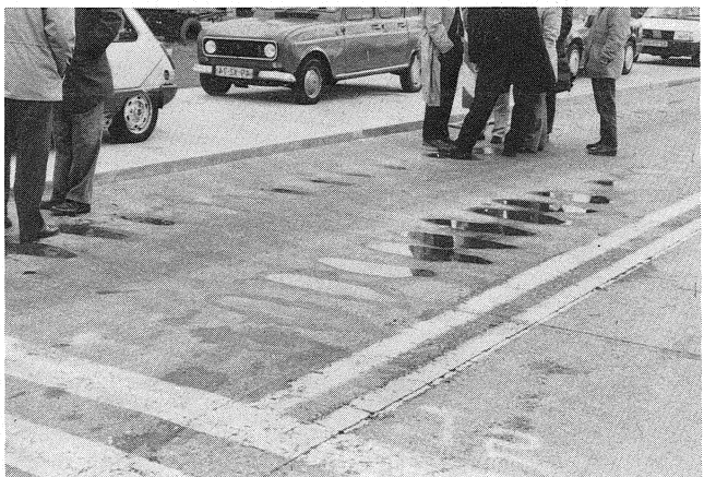
figure 1: Corrugation at a waiting lane
