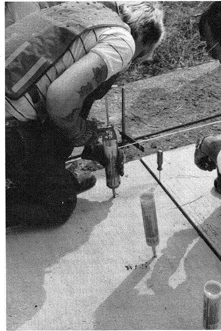
figure 6: Injection of the doweltube
