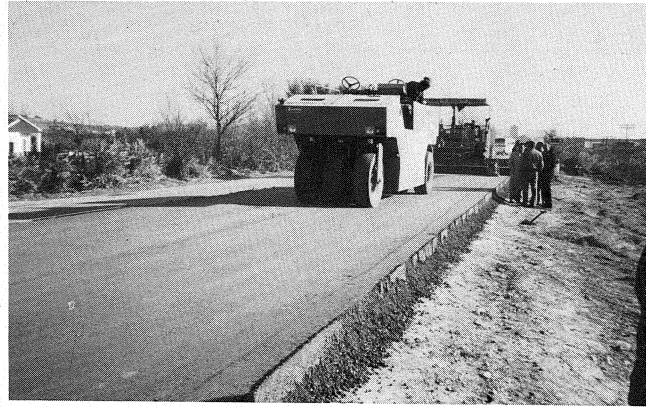
Fig. 11. Compaction with heavy rubber-tyred roller
