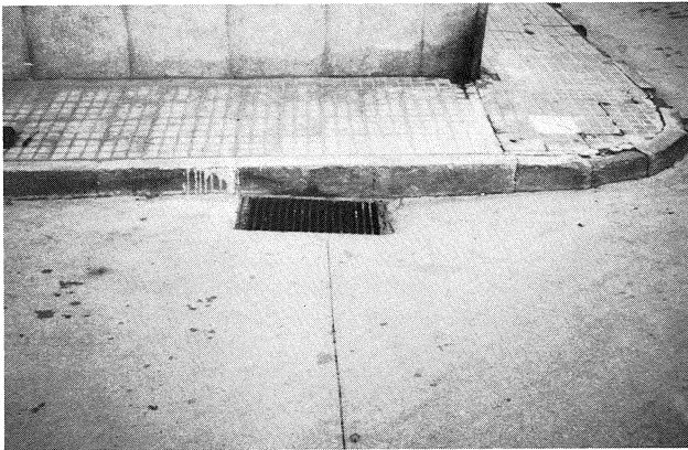
Fig. 6. RCC pavements for low volume roads: sawed joint
