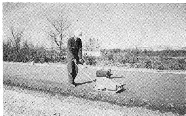
Fig. 12. Edge compaction with vibrating-plate
