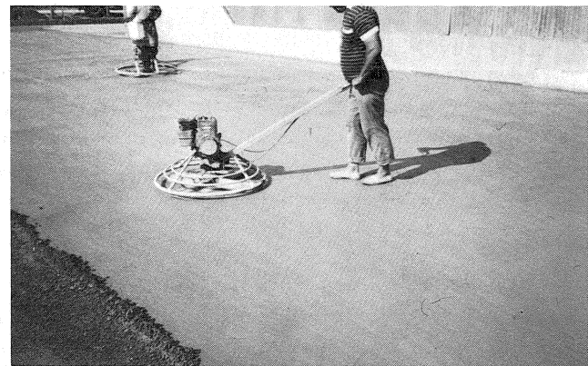
Fig. 4. Construction of RCC pavements for low volume roads: texturing with power trowels
