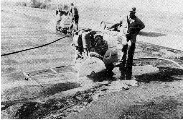
Fig. 14. Sawing of joints
