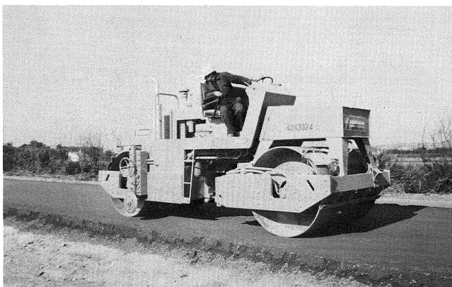
Fig. 10. Compaction with heavy smooth drum vibratory roller
