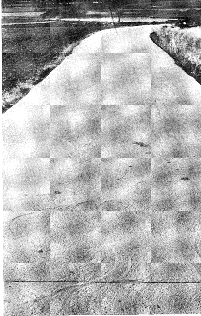
Fig. 5. RCC pavements for low volume roads: texture obtained through mechanical trowelling, and sawed joint
