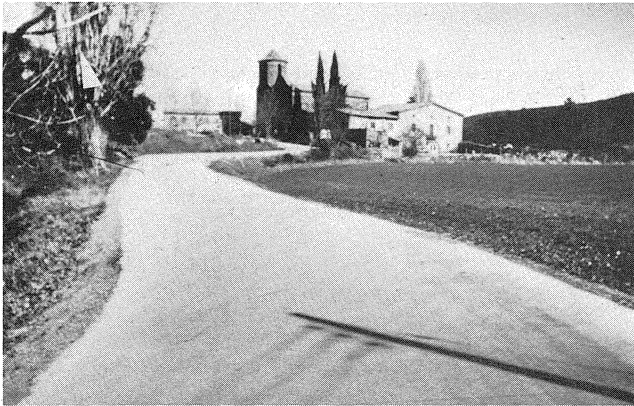
Fig. 1. Low volume road paved with RCC
