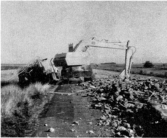
Figure 26. Magnet removing any residual from crushed concrete on I-90-94 project in Wisconsin.
