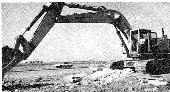
Figure 1. Note large size of concrete pieces being removed for disposal.
