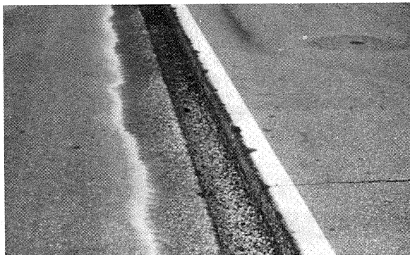
Figure 17. Edge drain has been placed 3' - 4' deep in existing asphalt surface prior to cold-milling the trench on this project on I-80.
