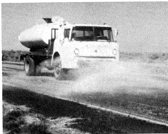
Figure 19. Spray wagon being used to cool asphalt surface prior to concrete placement on inlay project in Idaho.
