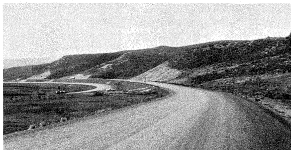
Figure 9. Asphalt surface after cold-milling and ready for concrete overlay on 1979-80 project in Utah.
