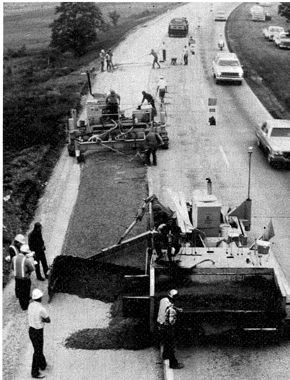
Figure 31. Tied concrete shoulder being added to existing pavement under traffic on I-81 in Pennsylvania.
