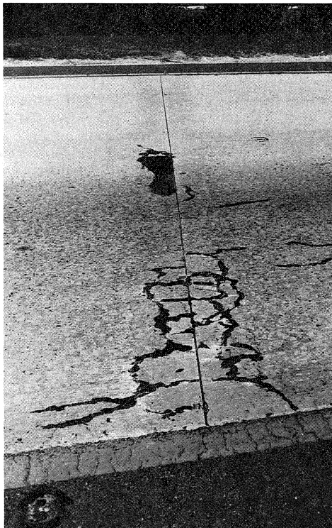
Figure 7. A failed joint with spalling, pumping and a punch out visible (condition rating 0,7).
