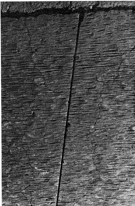
Figure 2. Development of small reaction cracks into load associated cracks (joint condition C = 0,5).
