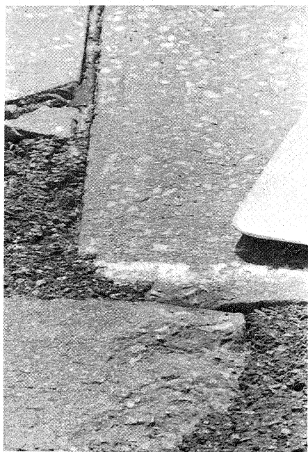
Figure 5. Transverse joint dislocation.
