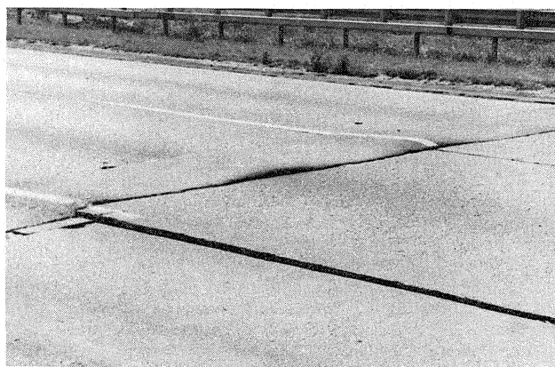
Figure 8. Transverse joint fault.
