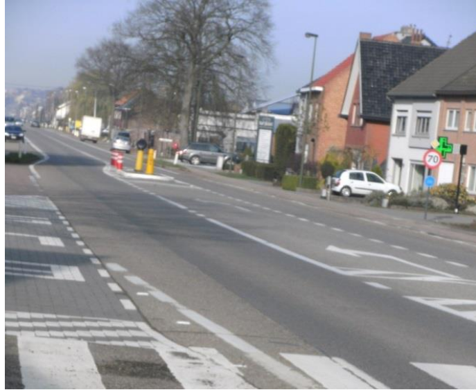
Figure 4. A CRC road, locally widened with concrete slabs
