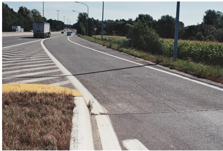
Figure 11 View at a locally widened CRCP by adding a triangle in CRCP
