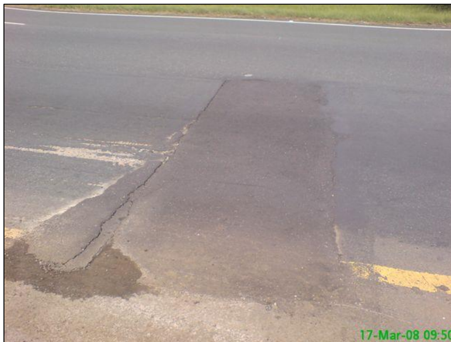
Figure 15: CRCP / Flexible Pavement Joint (N3/3, km 6.5 Southbound)
