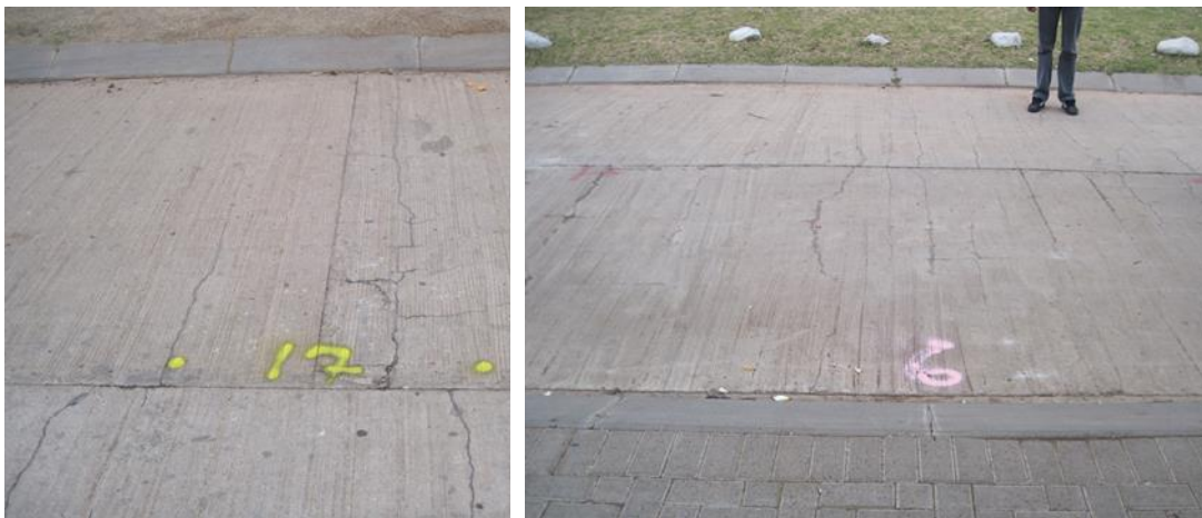
Figure 6: Traffic related early failures at the Mamelodi site
