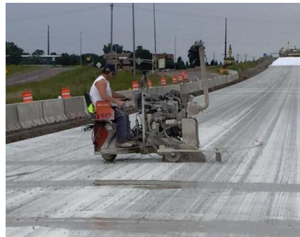
Figure 2. A typical conventional saw-cutting machine
