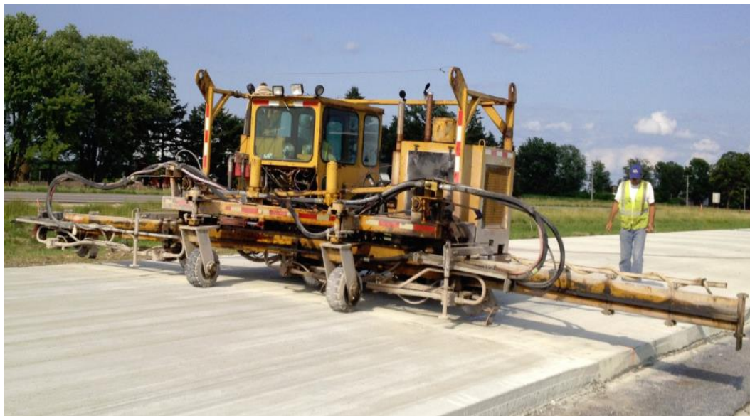
Figure 10. A span saw machine used at Site B
