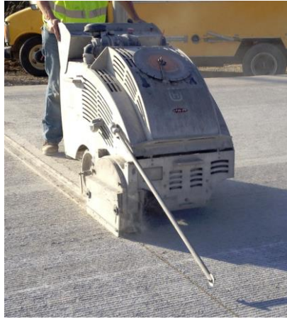
Figure 1. A typical early entry saw-cutting machine
