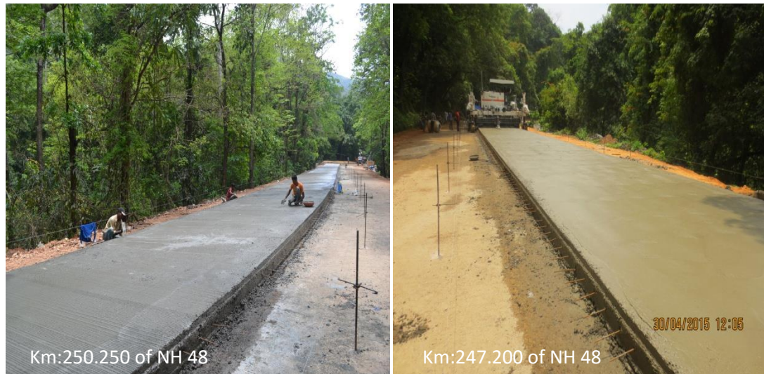
Figure 5 Photo Showing Stakes of Guide Wire Installed at Closer intervals
