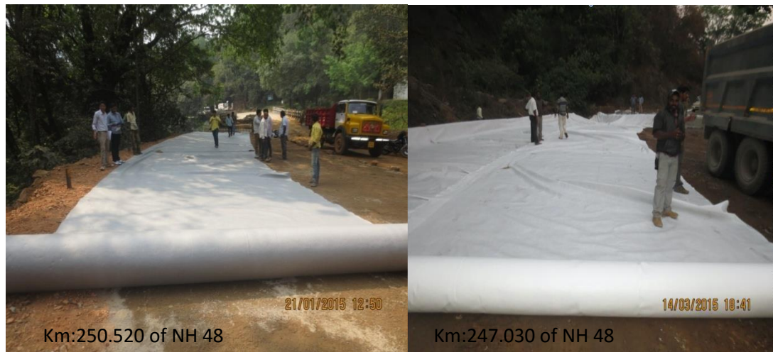
Figure 3 Laying of nonwoven Geofabric over the subgrade
