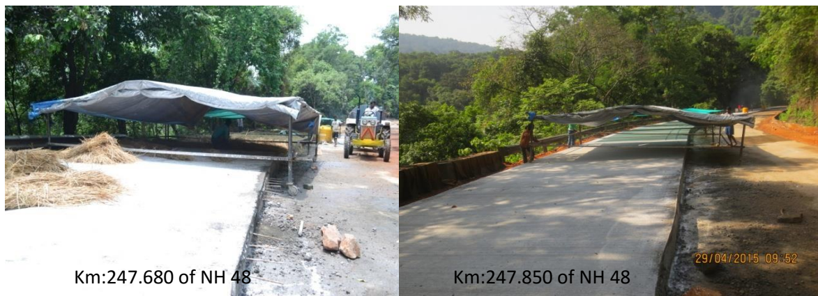
Figure 12 Temporary water proof Tent to CCP
