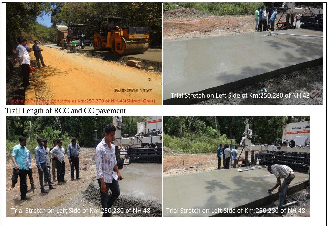
Figure 8 Trial of laying of cement concrete
