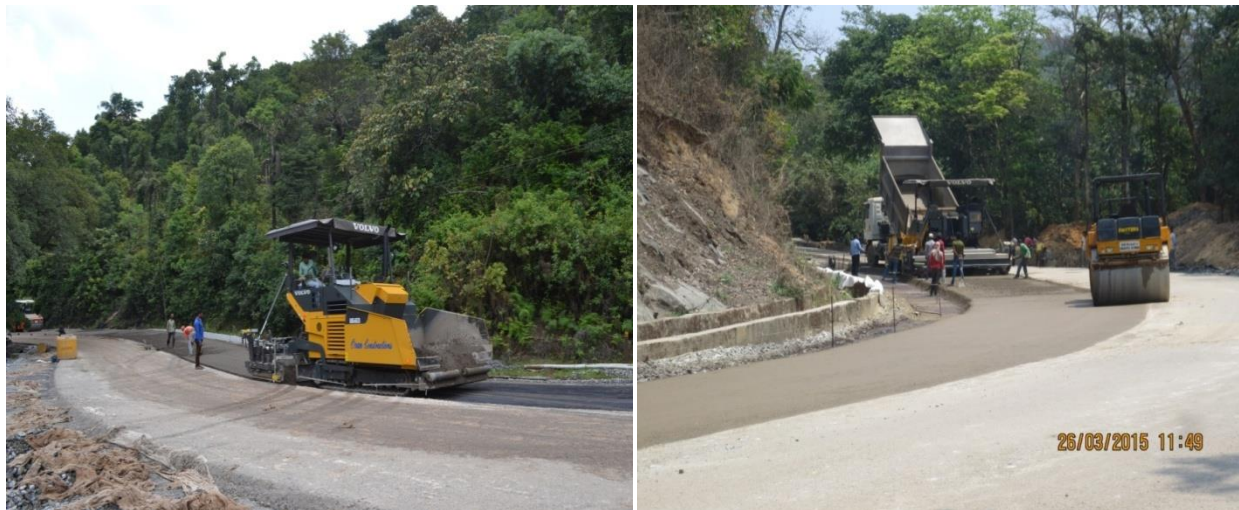
Figure 10 Showing the Laying of RCC at Km:246.720
