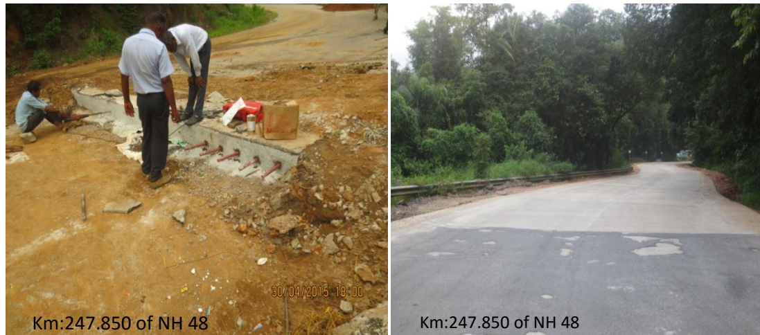
Figure 6. Dowel Bar insertion in the Existing pavement and new pavement to ensure Smooth ride quality
