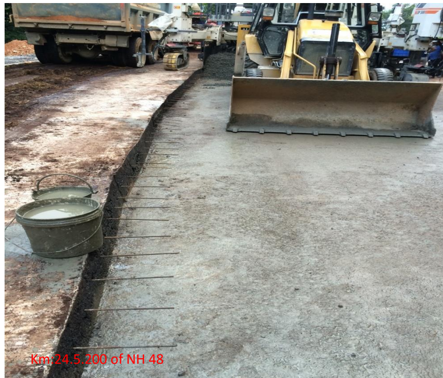
Figure 11 Applying Slurry Before laying of PQC
