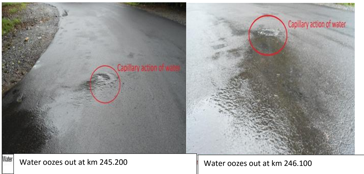
Figure 2 View of Artesian conditions
