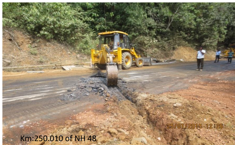
Figure 9 excavation of transverse furrow for drainage
