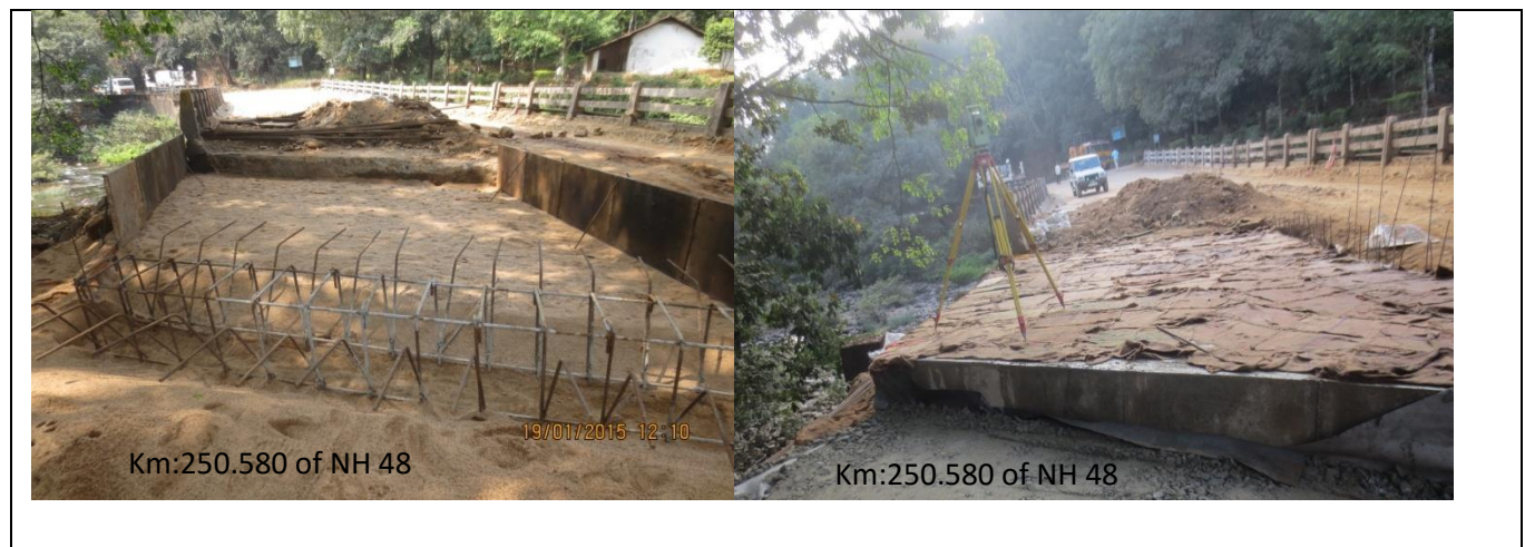
Figure 14 Photo of anchor beams constructed at site
