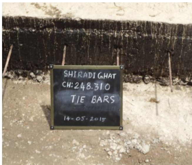
Figure 7 Fixing of Tie Bar with Epoxy Grouting
