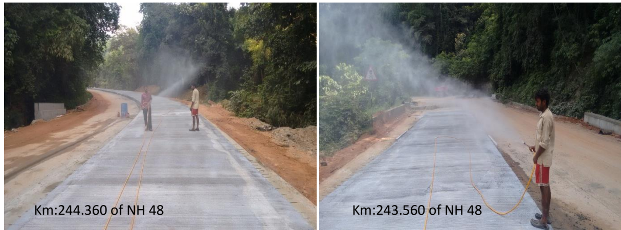
Figure 13 Mist Spray of water to prevent drying
