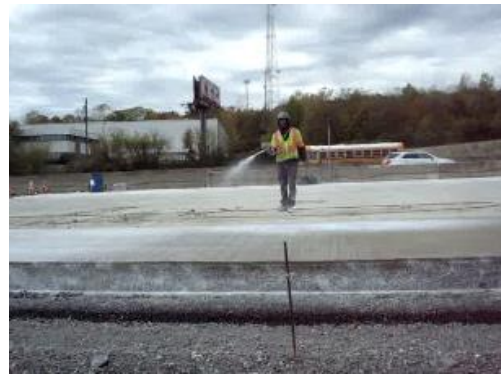
b. Curing compound application.
