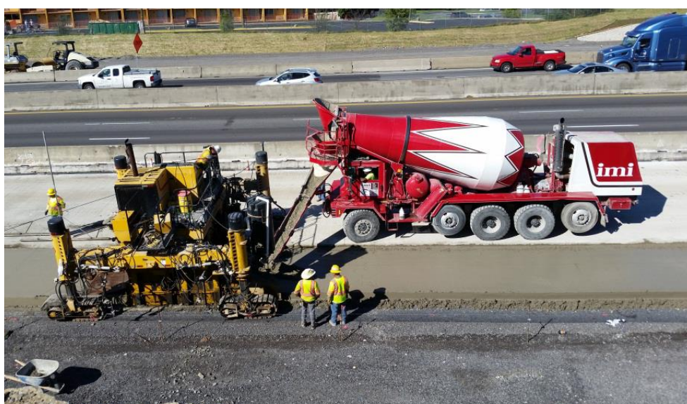
Figure 4. Top lift paving (photo courtesy of TDOT).
