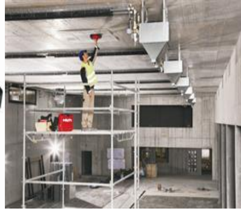
Figure7 (b): Scanner used to locate Rebars
