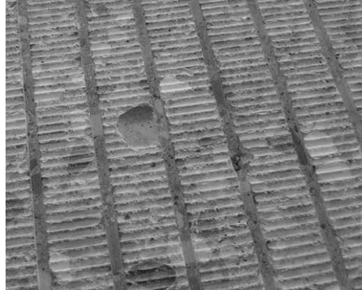
Figure 8. Example of coarse aggregate debonding due to deep grinding.
