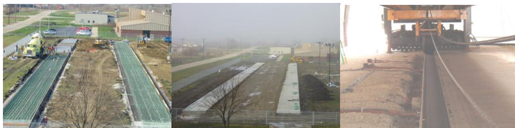
Figure 6.1: CRCP Test at ATREL, Rantoul, Illinois
