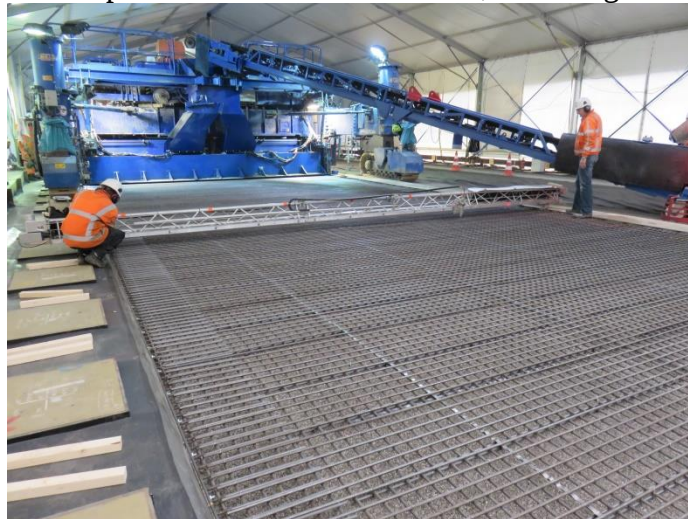
Figure 10 Front of the slipformpaver and in the front the reinforcement and the special developed ultrasound measurement system (Vissers, H.W.A.)
