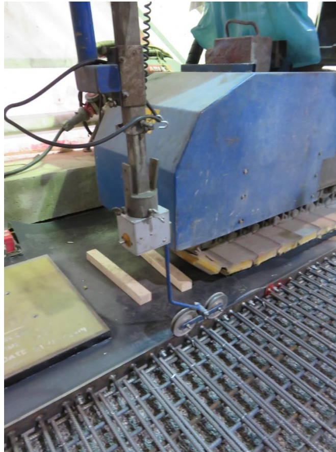
Figure 11 The electronic sensor for the driving direction of the slipformpaver (Vissers, H.W.A.).
