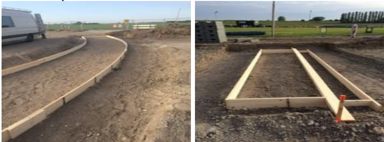
Figure 6a and 6b: Formwork for sleeper slab (l) and for connection concrete and asphalt
