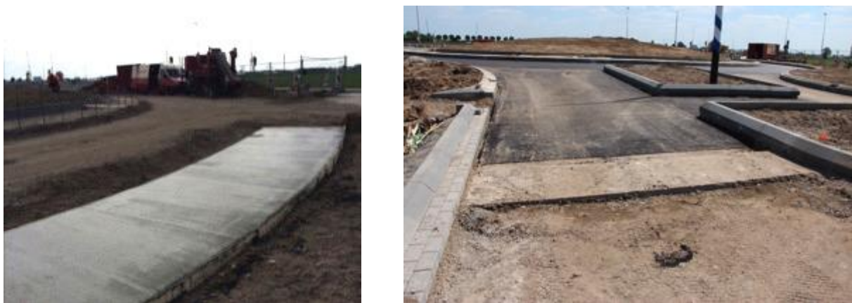
Figure 7a and 7b: Concrete for sleeper slab (l) and for connection concrete and asphalt
