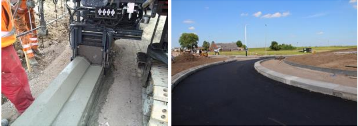
Figure 8a and 8b: slipformed concrete curb (RWS-type) and asphalt intermediate layer
