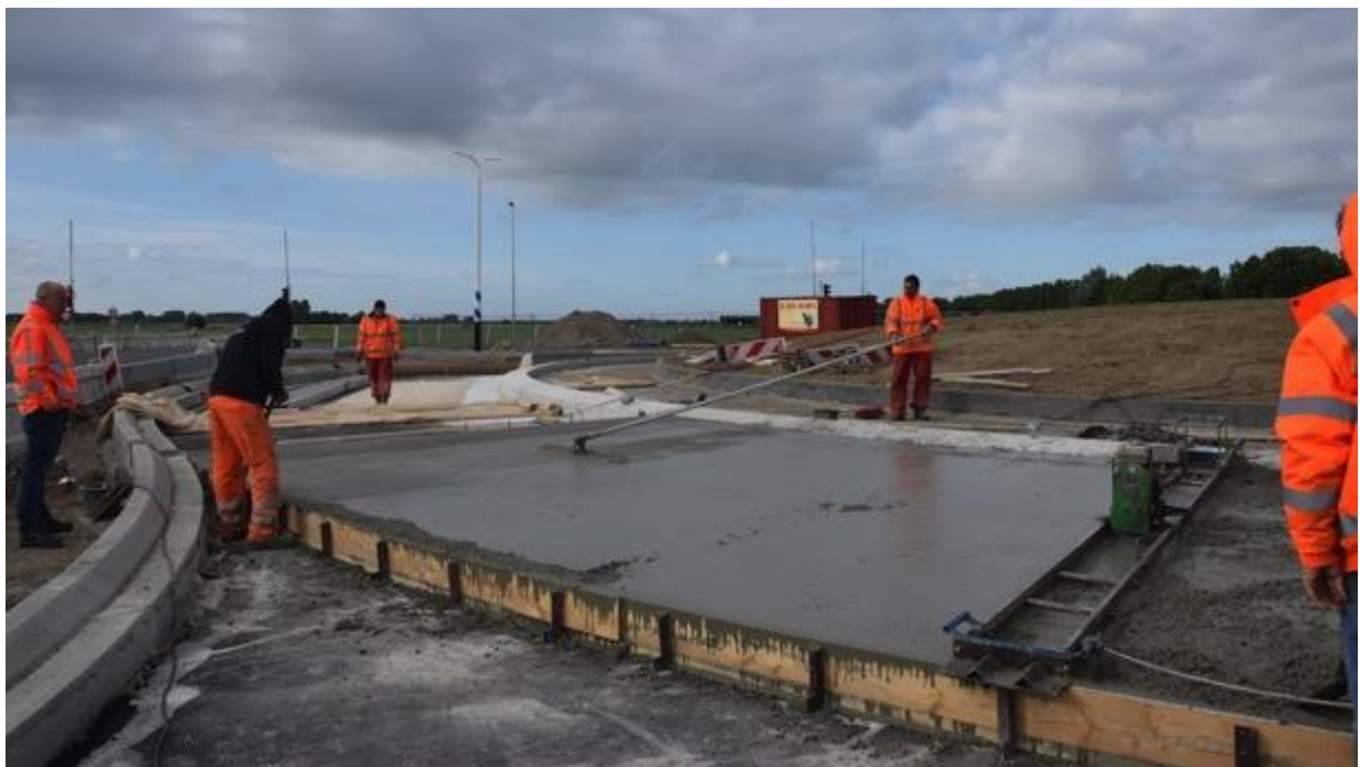
Figure 9: Manual application of concrete for roundabout
