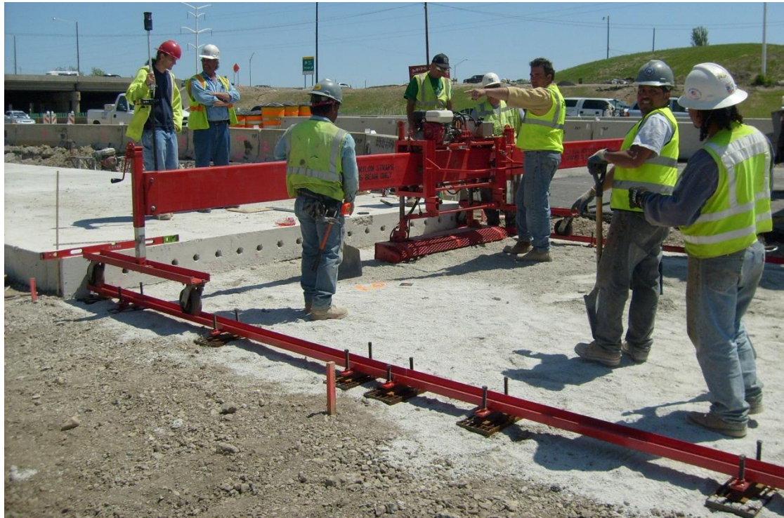
Figure 1: Large screed leveling base material (Source: Fort Miller Website (Fort Miller Compancy, Inc.))
