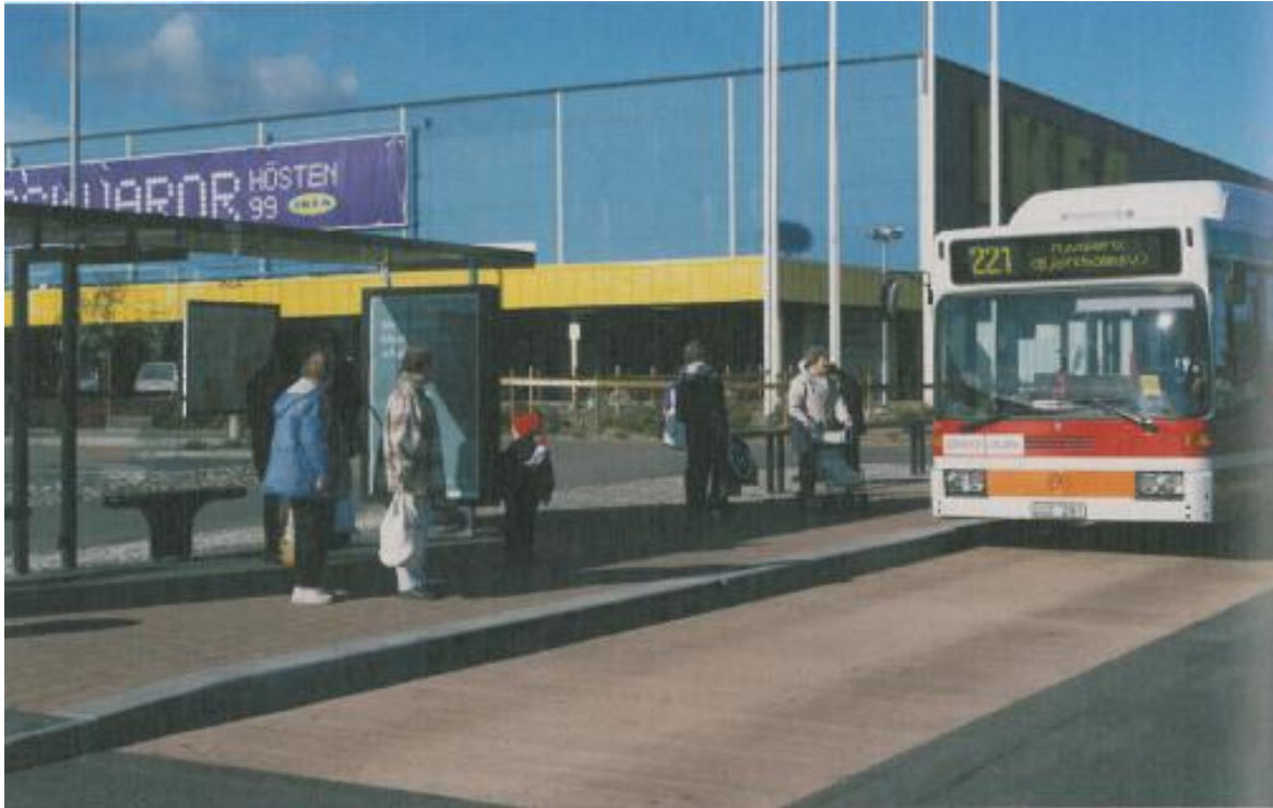
Figure 3 – Bus stop in Linköping, Sweden, area = 40 m 2 , thickness = 200 mm (Svensk Byggtjänst, 2002).
