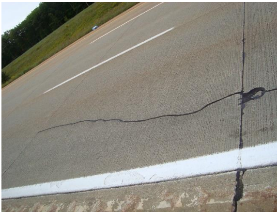
Figure 4: Random Longitudinal Crack, I-75 West Branch, Michigan
