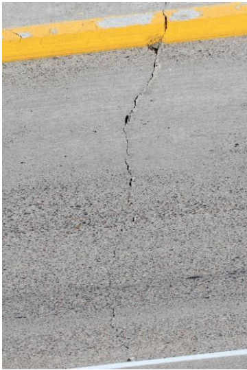
Figure 8: Reflective Transverse Crack at MnROAD Sub-Cell 405
