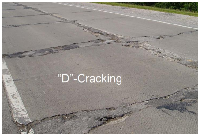
Figure 9: Condition of Route D in Missouri Prior To Overlay (Photo Courtesy of Todd LaTorella, ACPA)
